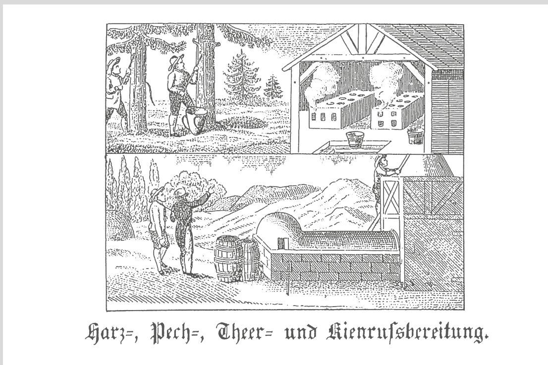
Figure 5: Processing pine resin to create pitch, tar and carbon black
