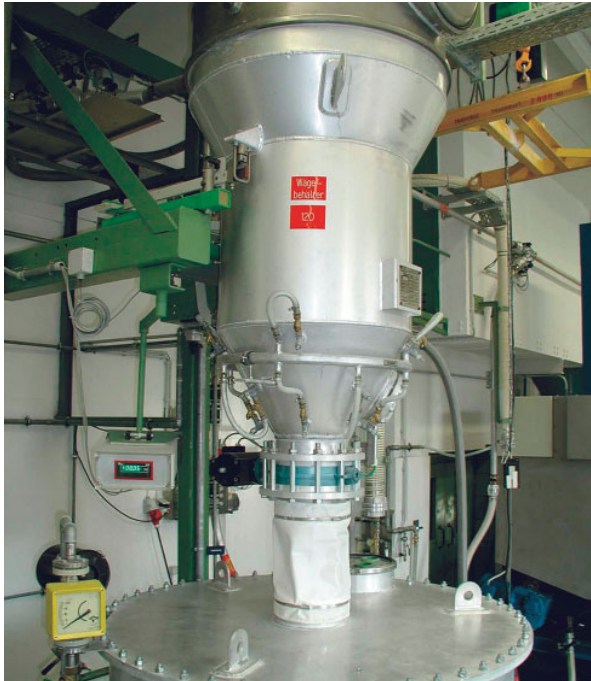
Container scale for batchwise metering
