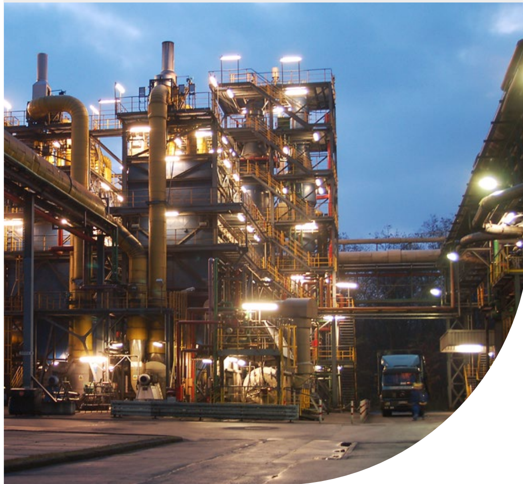
Orion's plant in Cologne, Germany.
