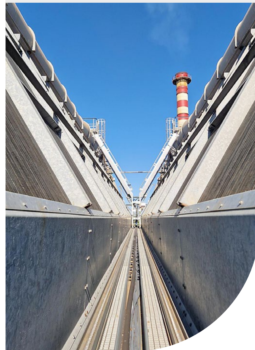
Orion's facility in Ravenna, Italy.
